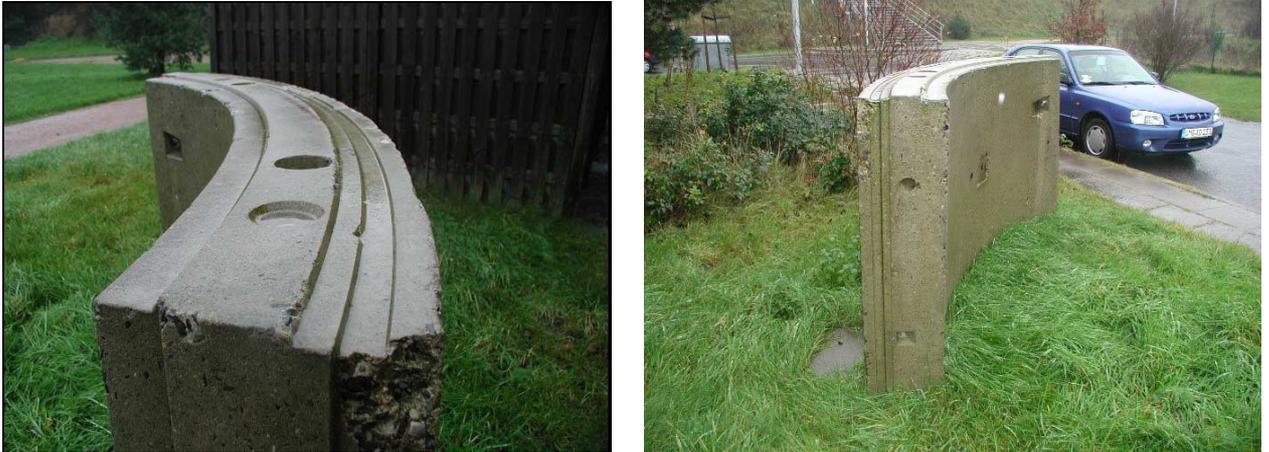
Figure 13: Concrete segments of the HERA tunnel.
