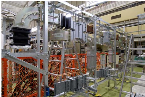
Linear distribution with circulator
