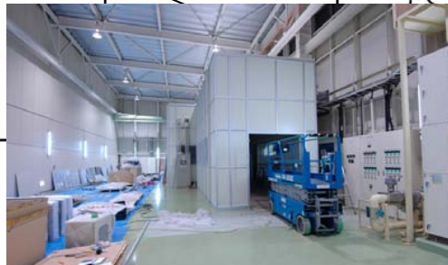
clean room construction
