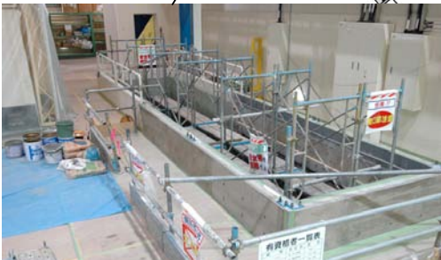
carry hatch expansion
